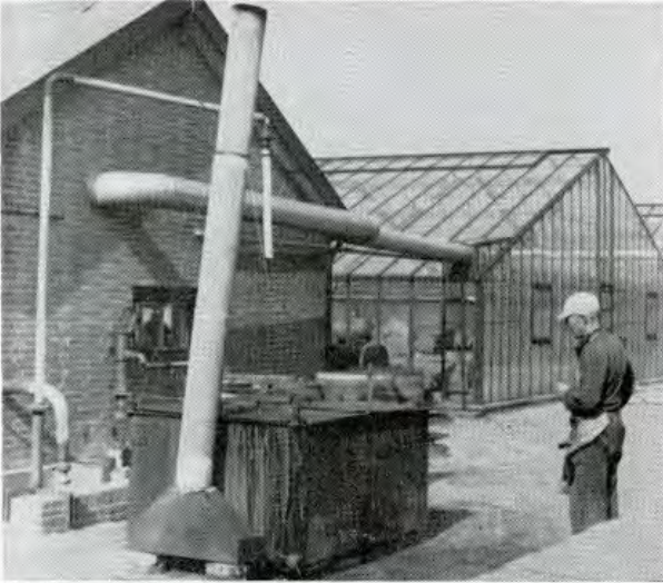
Fig. 22. UPPER , hot-water treatment of daffodil bulbs for killing nematodes.
